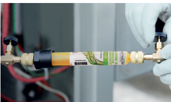
Charge inline with refrigerant
