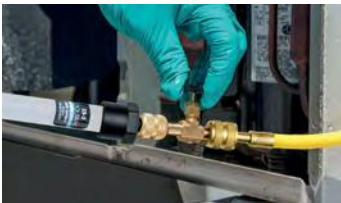
Charge inline with refrigerant
