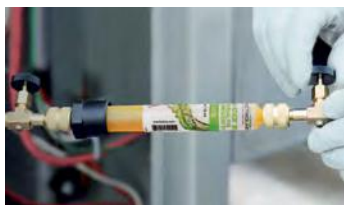
Charge inline with refrigerant
