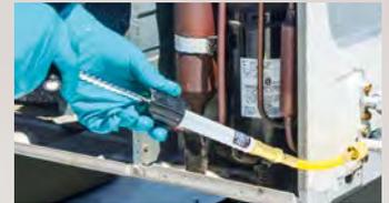
Inject dye with a turn of the handle.
