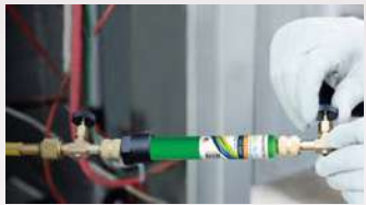
Charge inline with refrigerant
