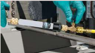
Charge inline with refrigerant
